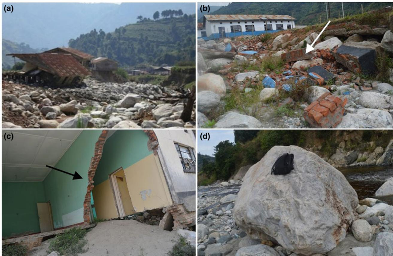
**Fig. 6** Examples of damage caused by the flood. **a** River bed and scour, **b** destruction of house foundation (*white arrow*), **c** destruction of house due to impact from debris (*black arrow*), **d** illustration of boulder size frequently found in the valley (backpack for scale)
