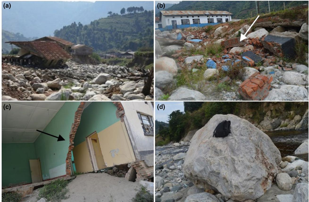
**Fig. 6** Examples of damage caused by the flood. **a** River bed and scour, **b** destruction of house foundation (white arrow), **c** destruction of house due to impact from debris (black arrow), **d** illustration of boulder size frequently found in the valley (backpack for scale)
