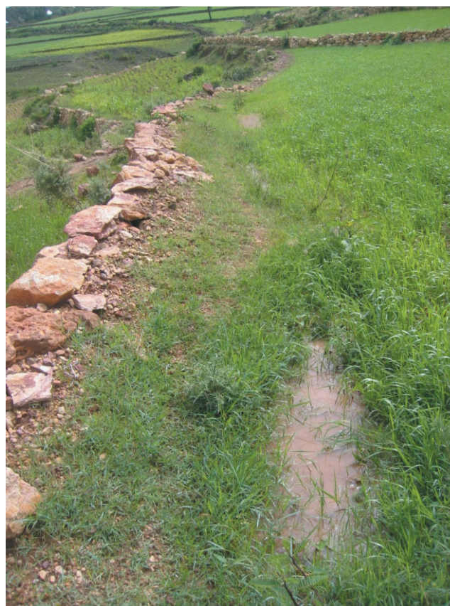
Figure 2. Stone bunds in the MZZ catchment induce retention of runoff (August 2006). This figure is available in colour online at www.interscience.wiley.com/journal/esp
